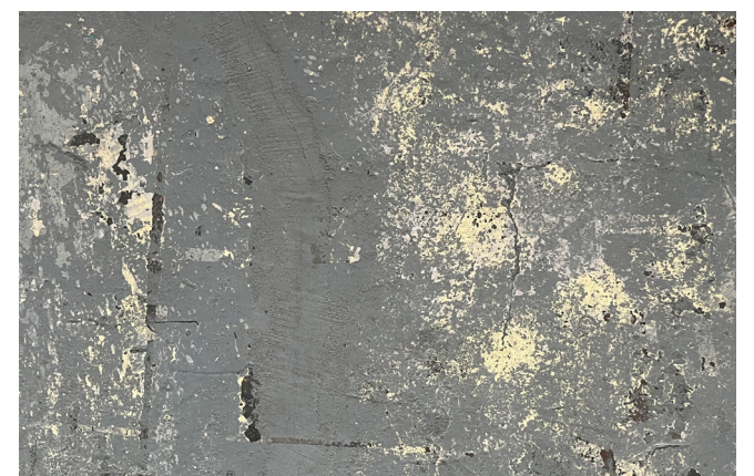
Betonboden S4 + S3
