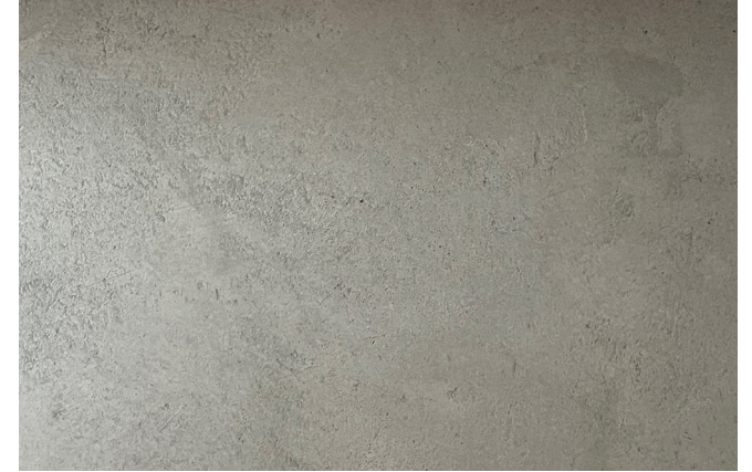
Concrete floor S1
