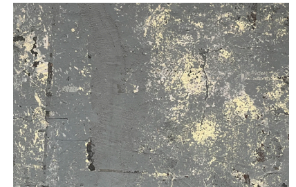
Industrial concrete floor
