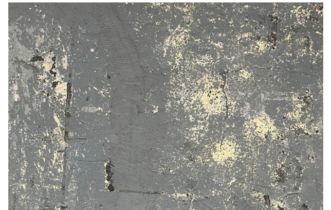
Concrete floor S4 + S3
